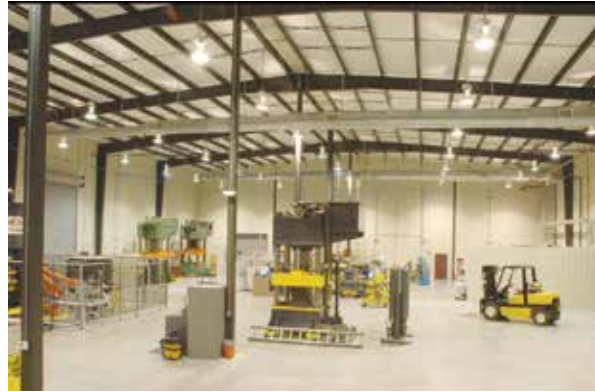
TYPICAL CONTINUOUS BEAM FRAME
